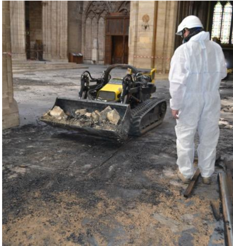
Cleaning operations by unmanned machines
