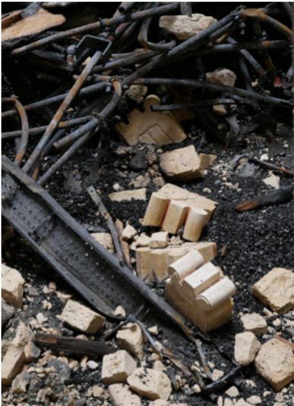
Voussoirs in the remains of the nave
