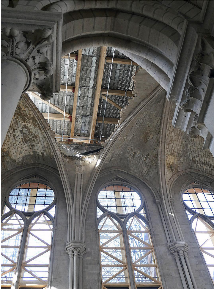
Collapsed arch (GT Pierre – Bruno Phalip)
